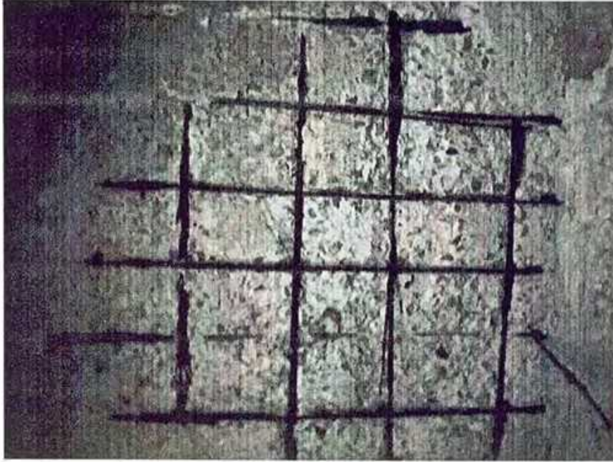
Photograph : Bottom surface of a slab
